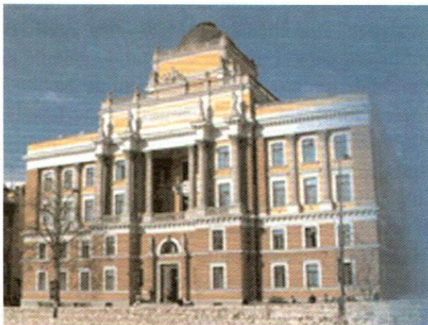
University of Sarajevo - Administration building
